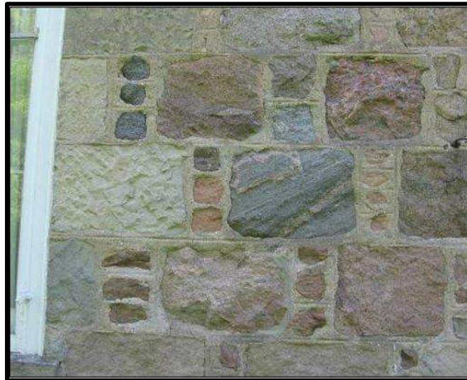
Figure 1: Example of Scottish Stonemasonry (Middleton 2011)
