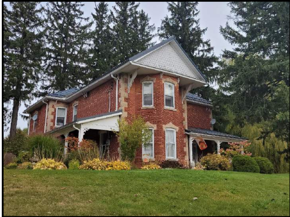
Image 10: South and West Elevation of 3 Station Street (Photo taken October 19, 2023; Facing Northwest)
