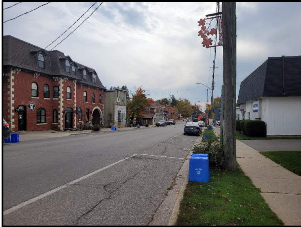
Image 9: Context View of Trafalgar Road Looking South (Photo taken on October 19,2023; Facing South)
