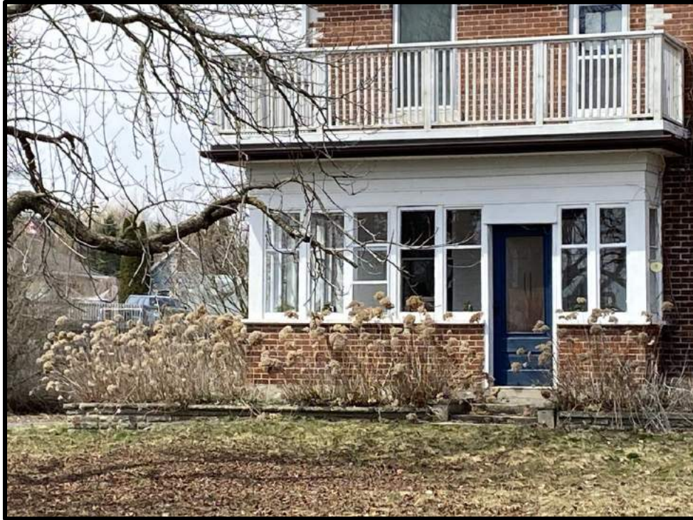
Image 7: Porch of 12 Orangeville Street (Photo taken on April 11, 2023; Facing North)
