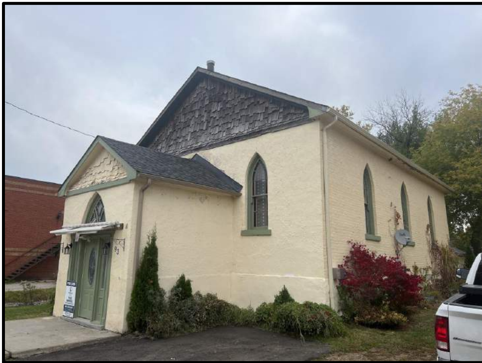
Image 8: Southwest Corner of 93 Trafalgar Road (Photo taken on October 19, 2023; Facing Northeast)
