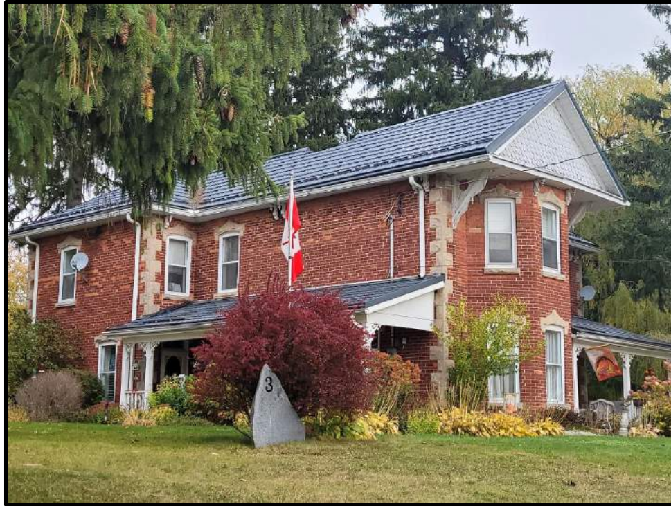
Image 11: West Elevation of 3 Station Street (Photo taken on October 19, 2023; Facing North)
