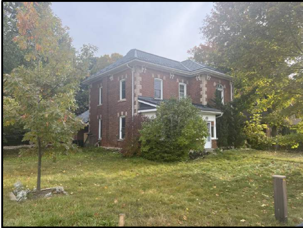
Image 7: Northwest Corner of 81 Trafalgar Road (Photo taken on October 19, 2023; Facing East)
