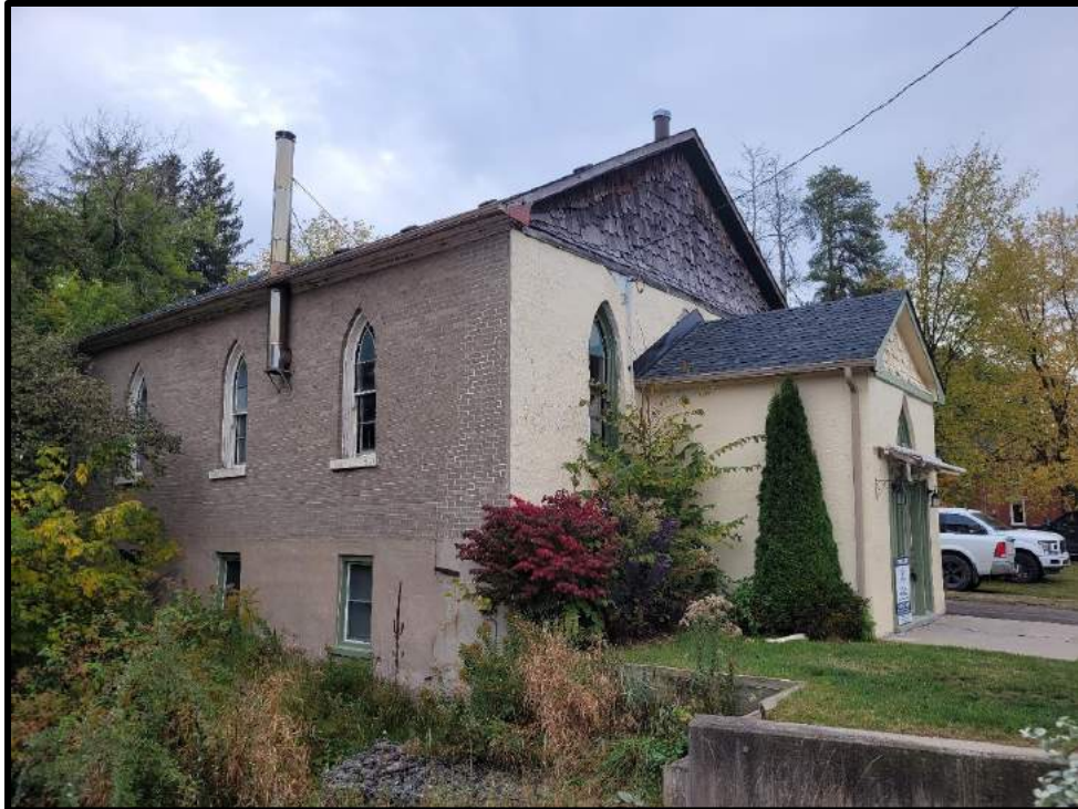
Image 5: Northwest Corner of 93 Trafalgar Road (Photo taken on October 19, 2023; Facing East)
