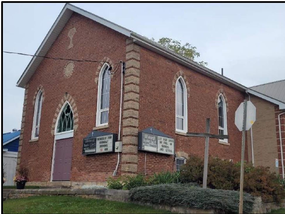
Image 8: Southwest Corner of 21 Trafalgar Road Showing Original Portion (Photo taken on October 19, 2023; Facing Northeast)
