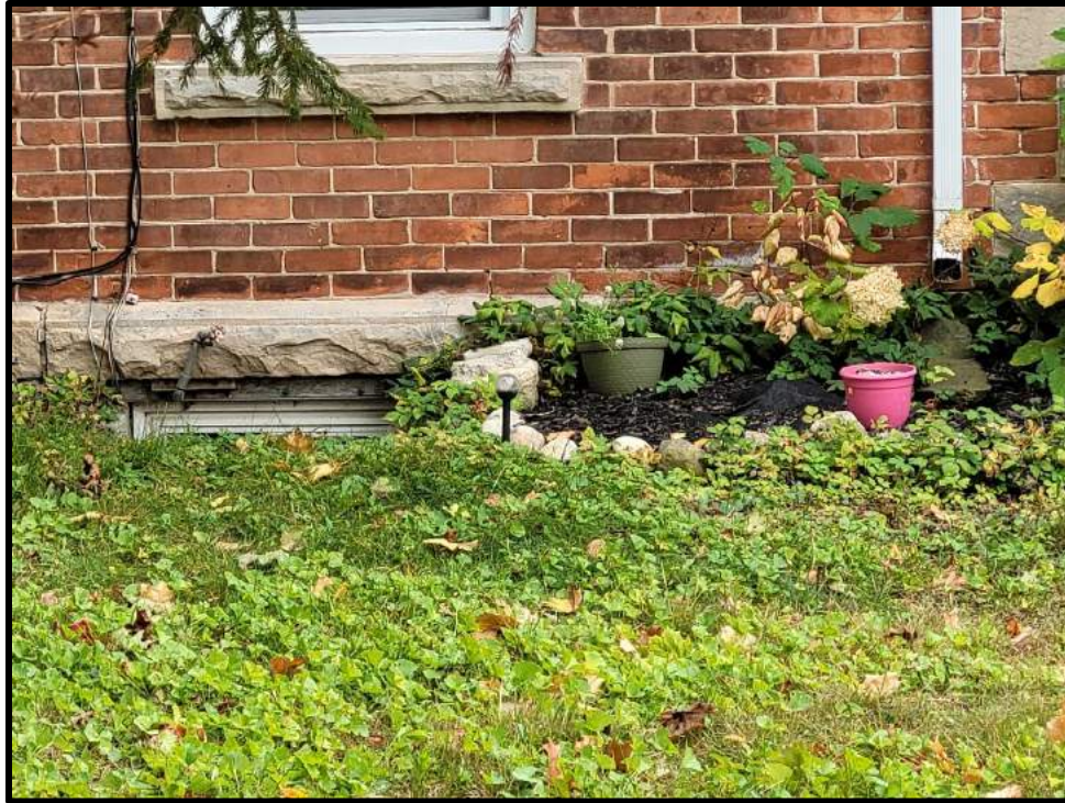
Image 5: Detail of Foundation of 81 Trafalgar Road (Photo taken October 19, 2023; Facing Northeast)
