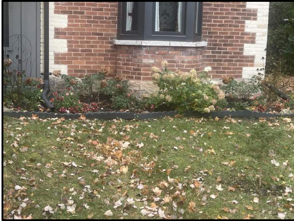
Image 5: Detail of Foundation of 114 Trafalgar Road (Photo taken on October 19, 2023; Facing West)
