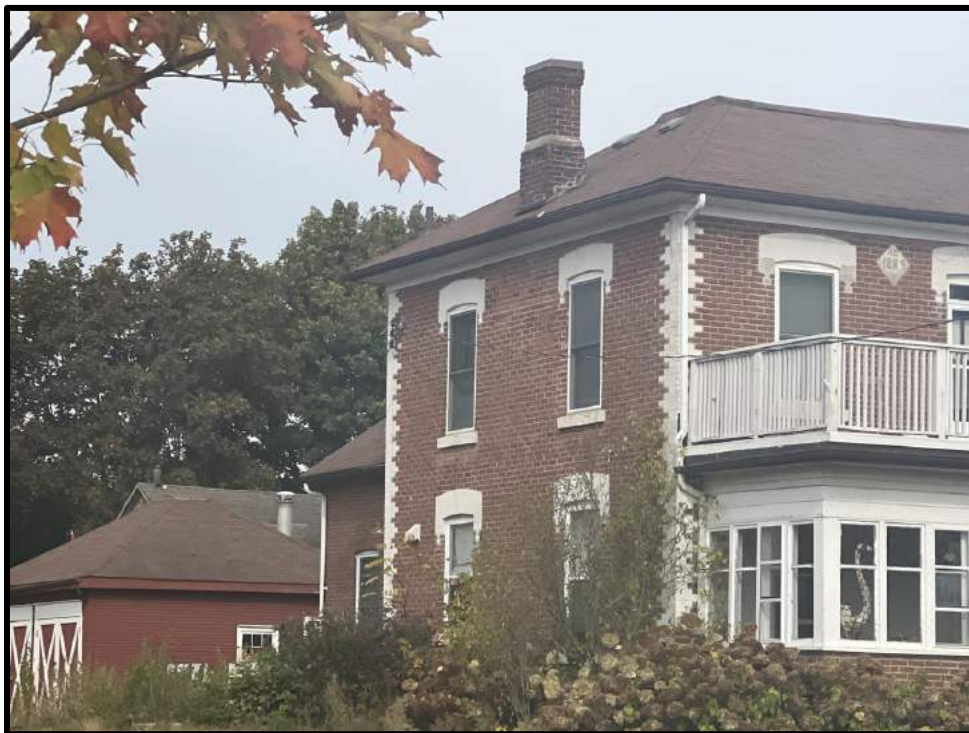
Image 6: West Elevation and Rear Garage of 12 Orangeville Street (Photo taken on October 19, 2023; Facing North)
