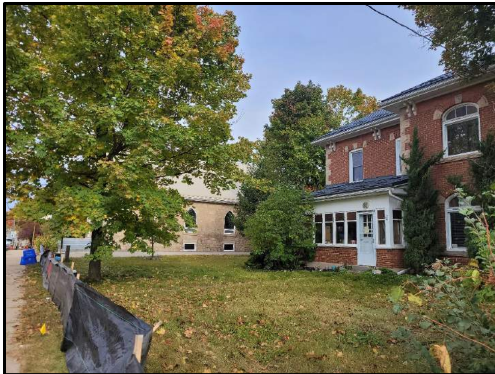
Image 13: View of 81 Trafalgar Road with Church in Background (Photo taken on October 19, 2023; Facing Northeast)
