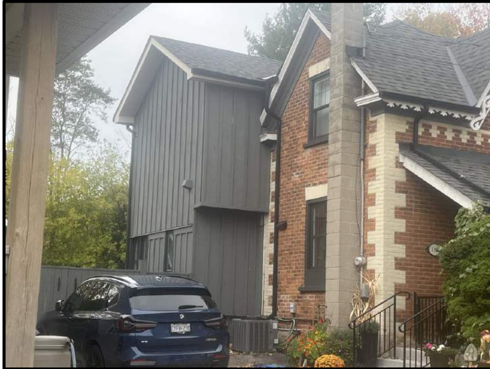
Image 8: South Elevation and Rear Addition of 114 Trafalgar Road (Photo taken October 19, 2023; Facing West)
