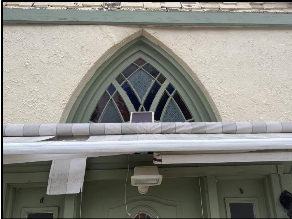
Image 3: Detail of Vestibule Window of 93 Trafalgar Road (Photo taken October 19, 2023; Facing Northeast)
