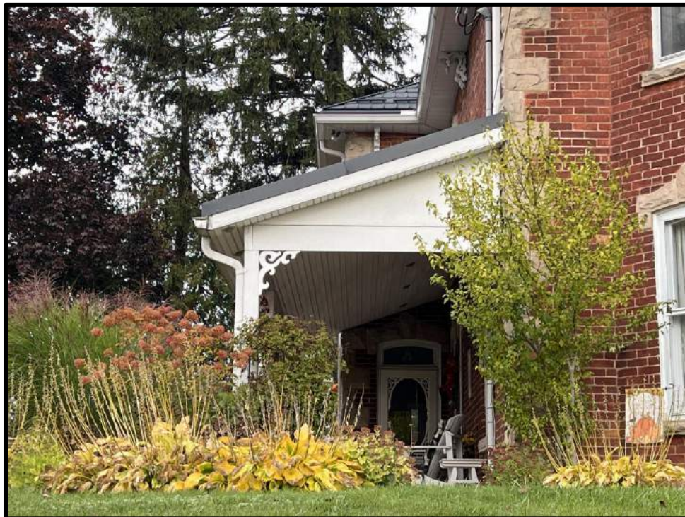
Image 4: Detail of Side Porch and Entranceway on West Elevation of 3 Station Street (Photo taken October 19, 2023; Facing Northwest)
