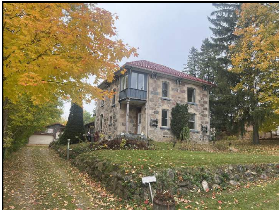
Image 4: South Elevation of 18 Anne Street (Photo taken October 19, 2023; Facing West)
