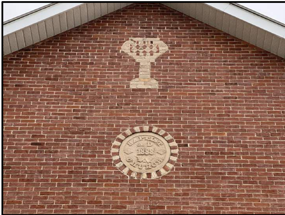
Image 2: Detail of Date Stone and Brick Chalice on Façade of 21 Trafalgar Road (Photo taken October 19, 2023; Facing Northeast)
