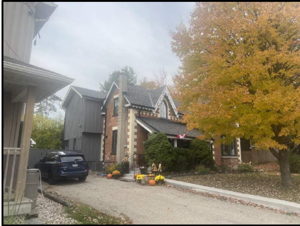
Image 7: Southeast Corner of 114 Trafalgar Road (Photo taken October 19, 2023; Facing West)
