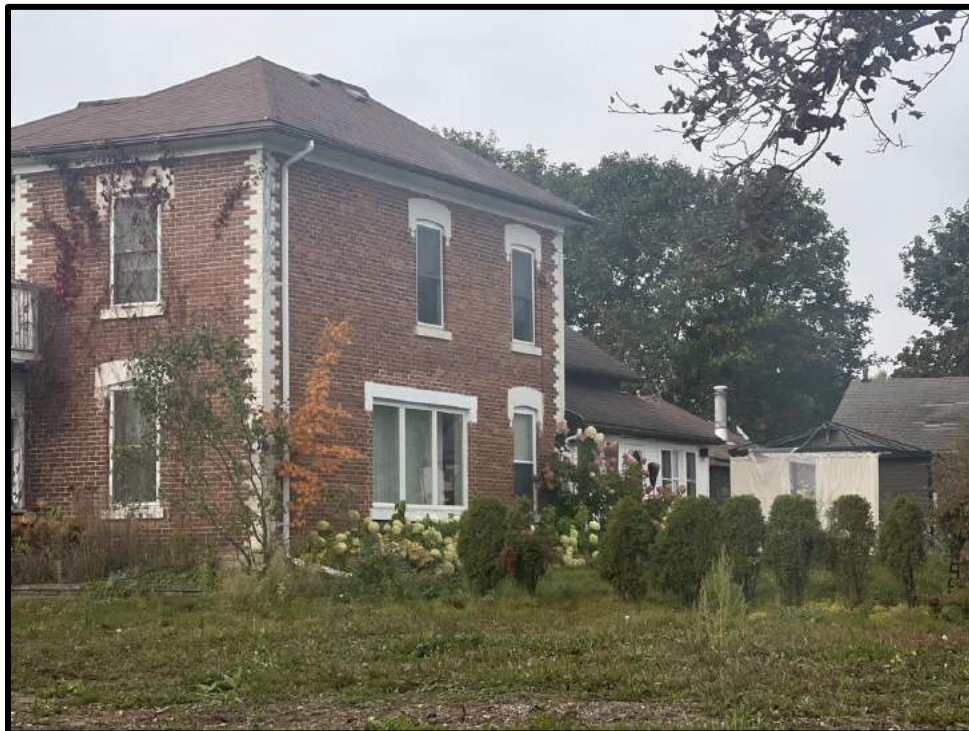
Image 4: View of East Elevation and Rear Addition of 12 Orangeville Street (Photo taken October 19, 2023; Facing Northwest)
