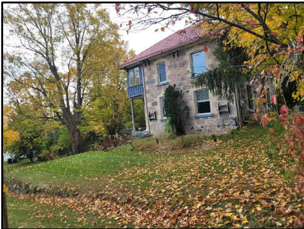
Image 6: View Stone Retaining Wall of 18 Anne Street (Photo taken on October 19, 2023; Facing South)
