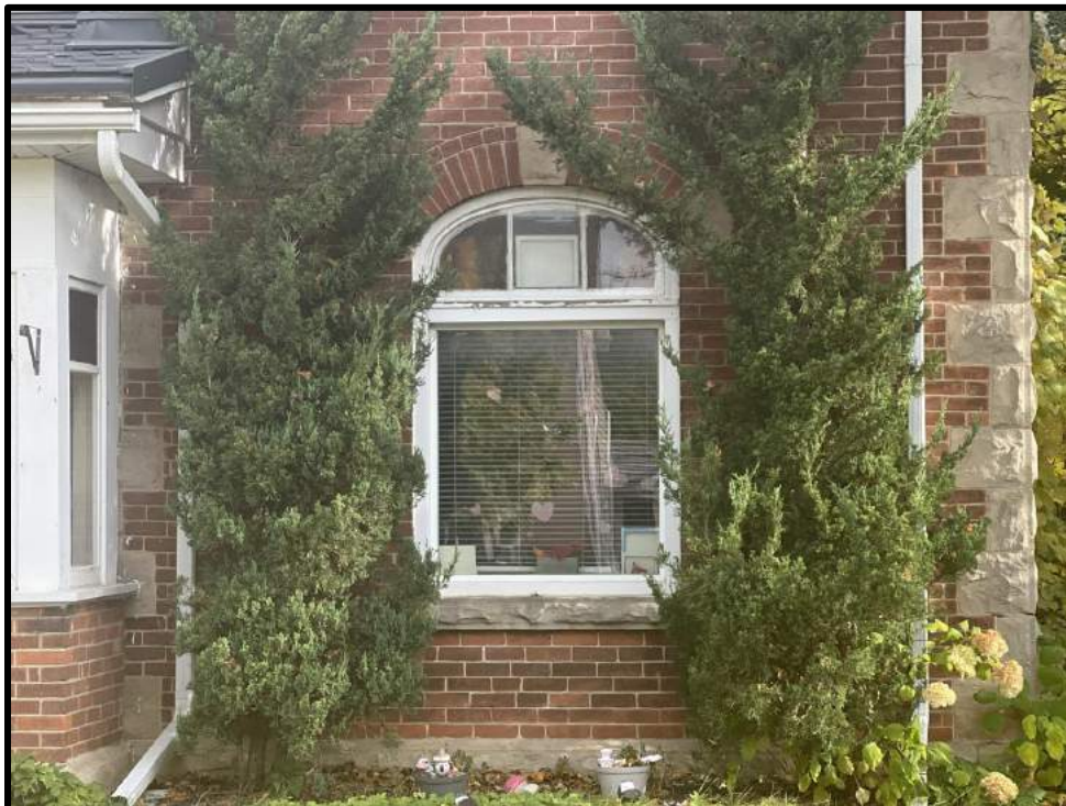
Image 2: Detail of Elliptical Arch Window Opening of 81 Trafalgar Road (Photo taken October 19, 2023; Facing Northeast)
