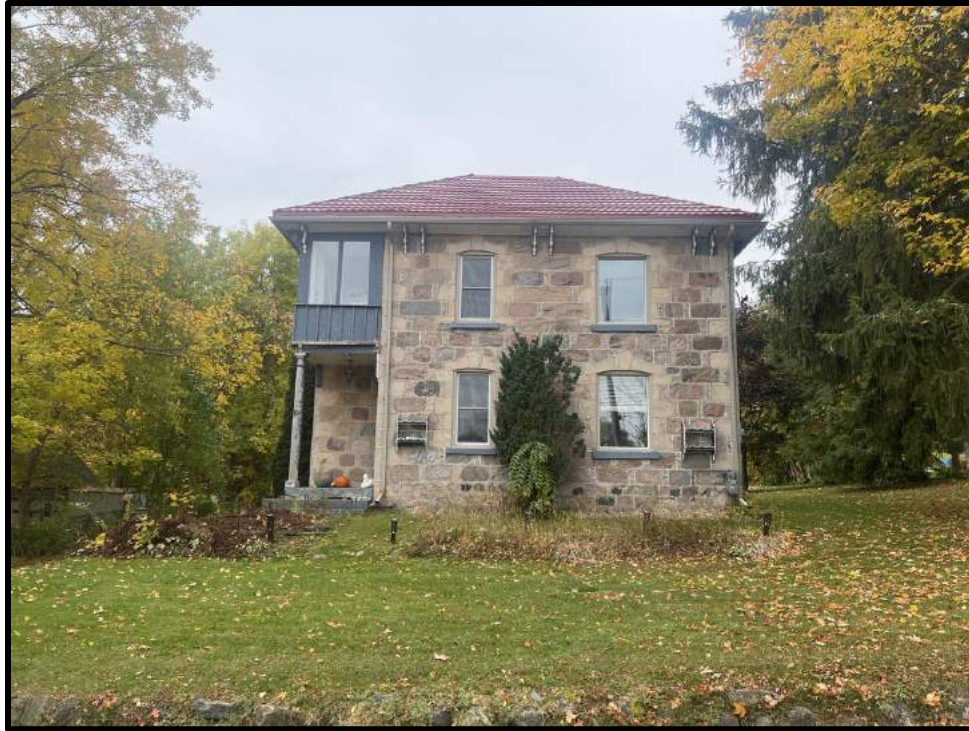
Image 1: Façade of 18 Anne Street (Photo taken October 19, 2023; Facing Southwest)
