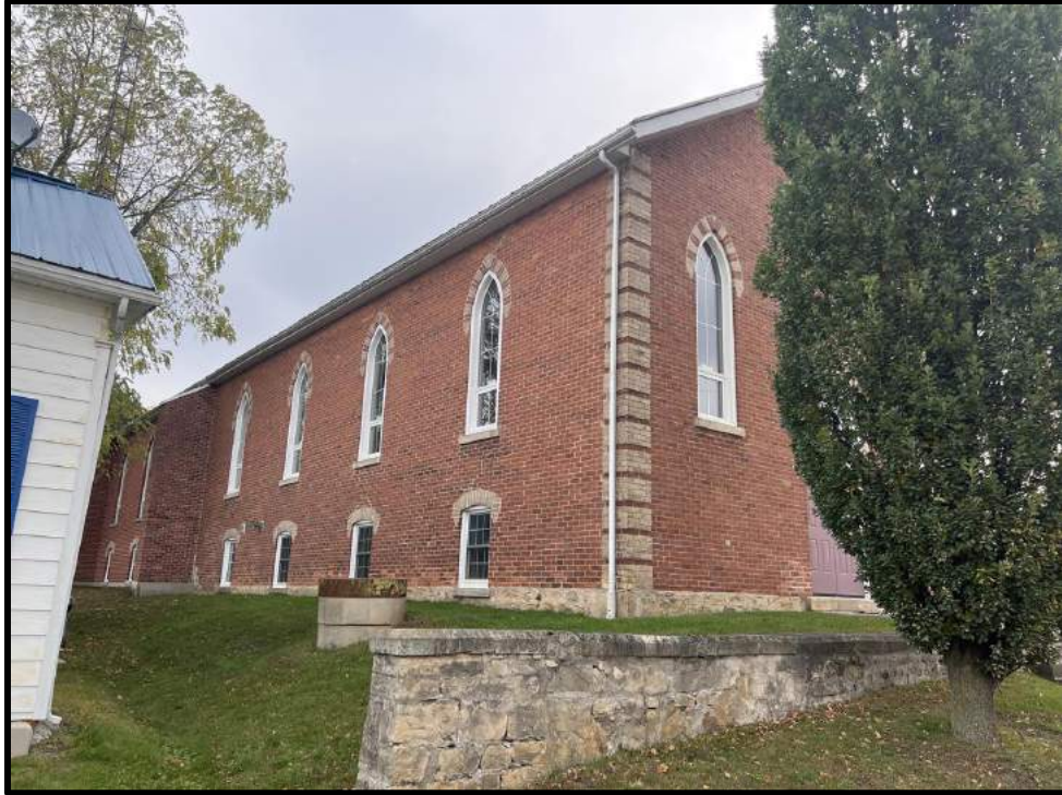
Image 7: Northwest Corner and Retaining Wall of 21 Trafalgar Road (Photo taken on October 19, 2023; Facing Southeast)
