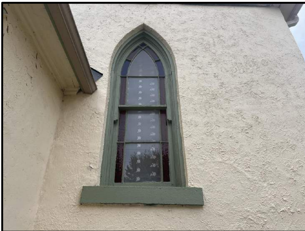
Image 4: Detail of Lancet Window Opening of 93 Trafalgar Road (Photo taken October 19, 2023; Facing Northeast)
