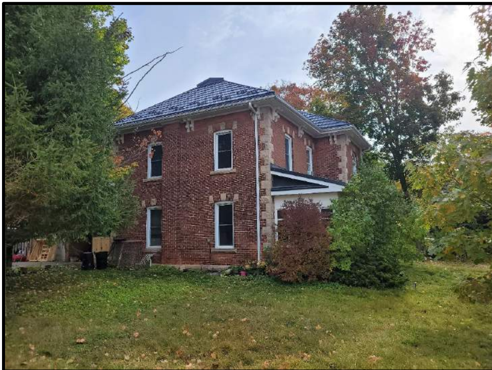
Image 8: North Elevation of 81 Trafalgar Road (Photo taken on October 19, 2023; Facing East)
