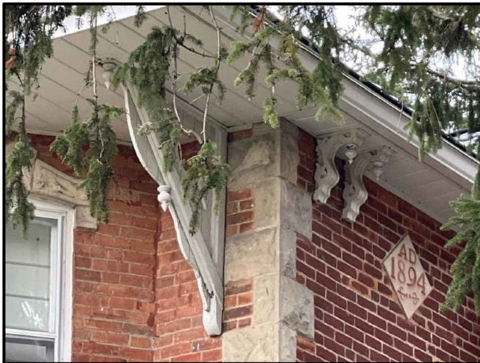
Image 6: Detail of Date Stone and Wood Brackets of 3 Station Street (Photo taken on October 19, 2023; Facing West)
