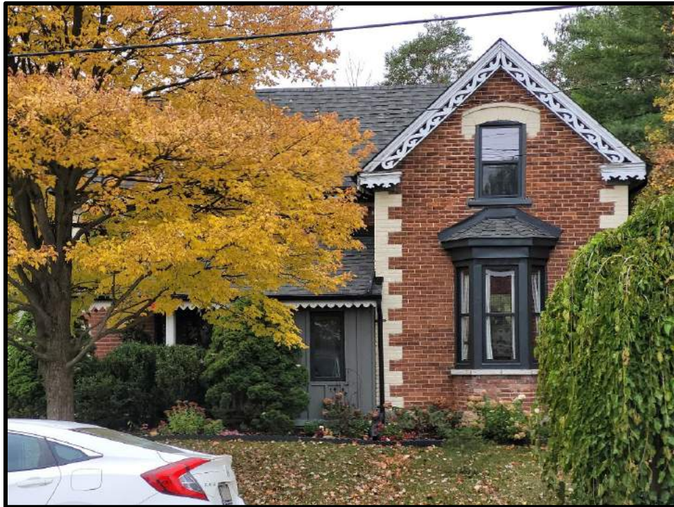
Image 6: Detail of Bay Window of 114 Trafalgar Road (Photo taken October 19, 2023; Facing West)
