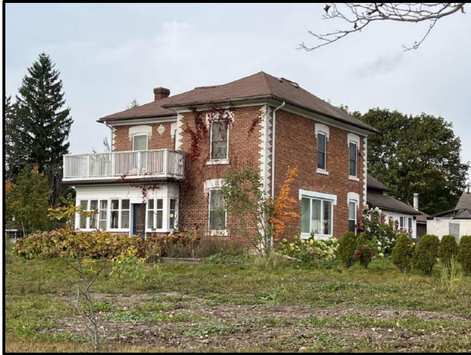
Image 3: Southeast Corner of 12 Orangeville Street (Photo taken October 19, 2023; Facing Northwest)
