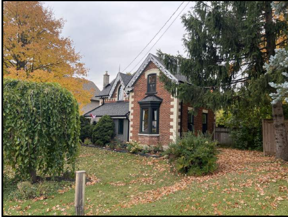
Image 3: Northeast Corner of 114 Trafalgar Road (Photo taken October 19 ,2023; Facing Southwest)
